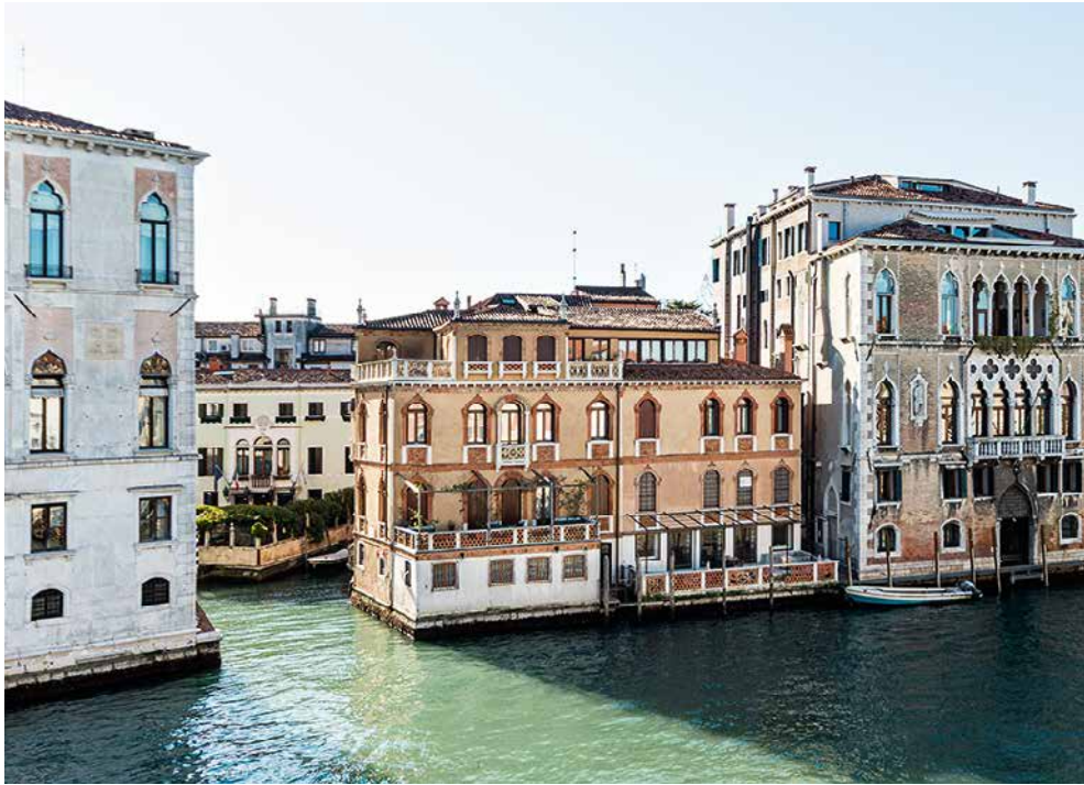
1 View of Ca' Marioni-Mainella on the Grand Canal. Casa Balboni is in the right-hand side of the building, on the ground and first floors.
